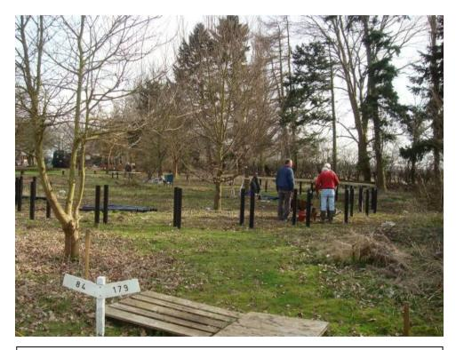
Work is now underway again on the new "G1" track. In the foreground Matt Stallard, David Wesy & Norman Back are busy filling the pipe with concrete and setting the top studding. Geoff Mogg is at the back checking laser levels are correct.
